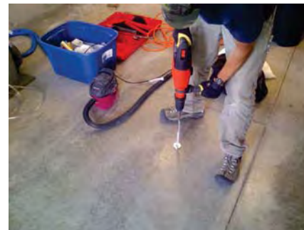
Installation of a Sub-Slab Soil Vapor Pin
