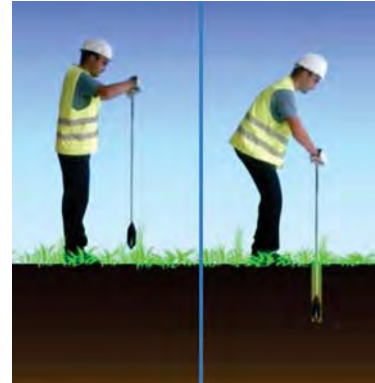
Installation of a Source Area or Near-Slab Soil Vapor Well
